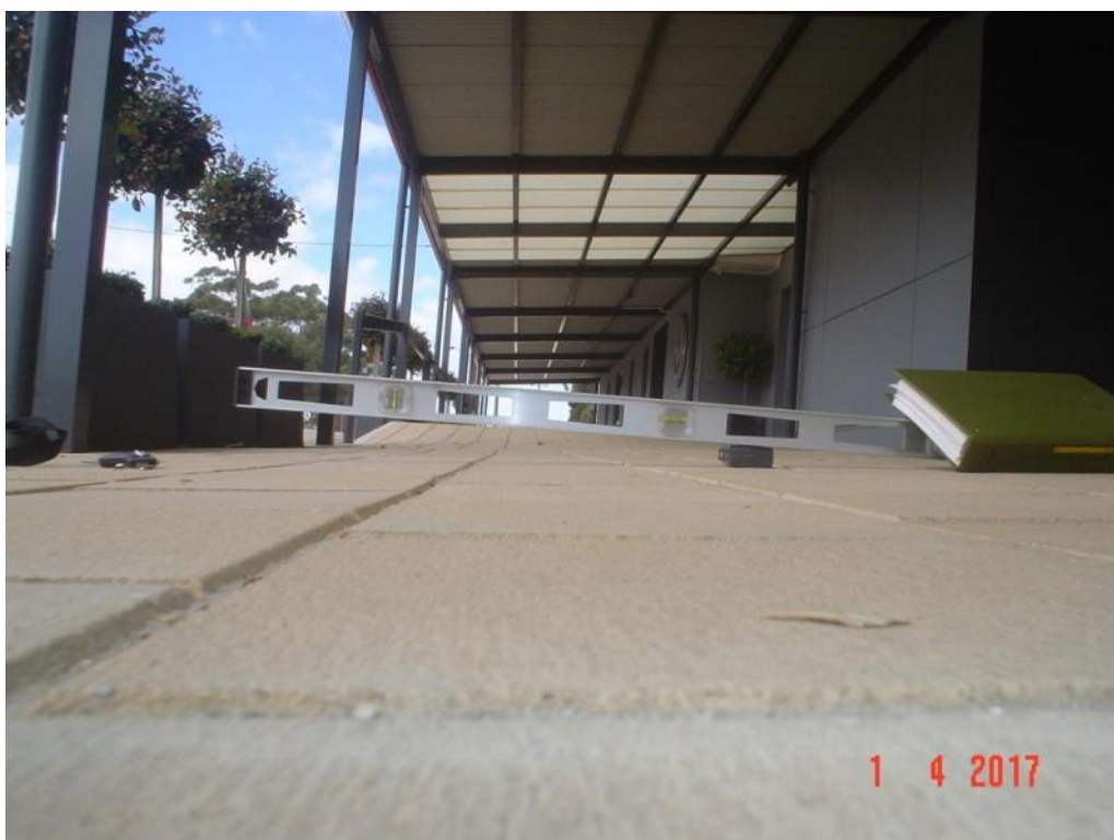
Plate 12 Crossfall downhill from the main door (1:16, 6.3%)
