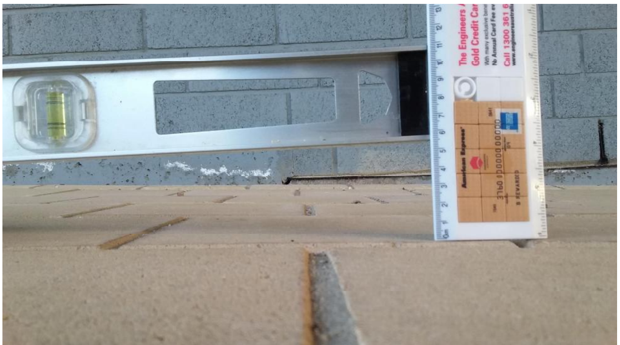
Plate 6 Longitudinal fall downhill from the corner of building (1:21, 4.8%);
