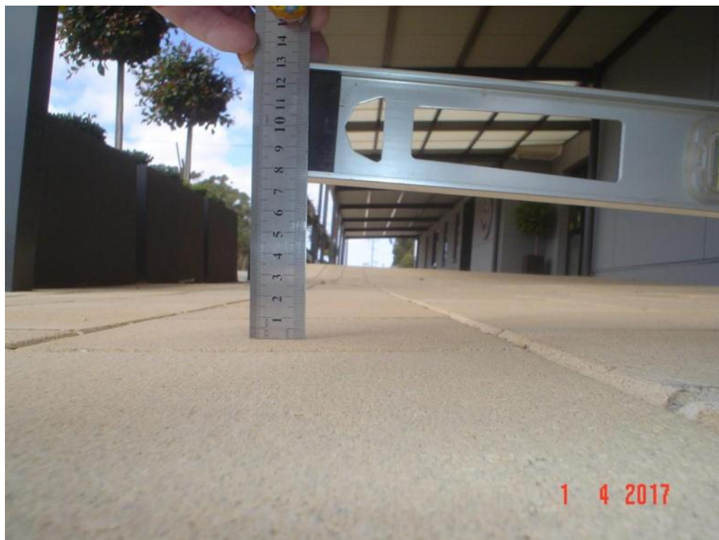
Plate 13 Crossfall 76mm in 1220mm down from the main door. (1:16, 6.3%)
