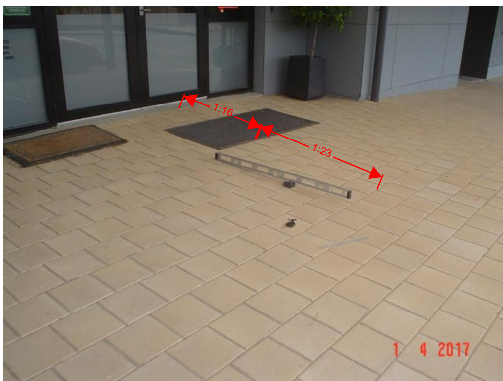
Plate 8 Measuring the crossfall in front of main entrance (1:23, 4.3%)
