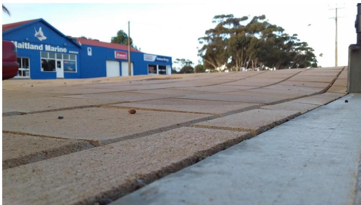
Plate 2 Egress from disabled parking (No landing for the change of direction)
